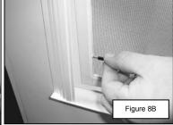
**D.** Pull the two retractable screen pins towards each other, then rotate the screen into place and push screen so it rests on top of bottom screen.
