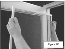
**C.** To remove the screen(s), pull the two screen pins toward each other then pull them toward you. Rotate the screen out of its track.
